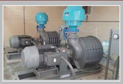
The City of Webster recently installed new blowers at their wastewater treatment plant. Needing to upgrade from aging technology, the City installed two 150 HP multistage centrifugal blowers by Continental Blower. The engineering design was done by Freese and Nichols (Pearland) and the blowers were installed by Sustanite Support Services (Houston).
