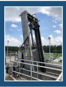
The City of Houston recently awarded a project to rehabilitate their Suez Climber Mechanical Bar Screen at their Kingwood WWTP. The project was set up on a turnkey basis whereby the rake mechanism and cogwheel pin racks were removed and replaced with new components. We have handled many rehabilitations of this type of coarse screen as well as other fine screens.
